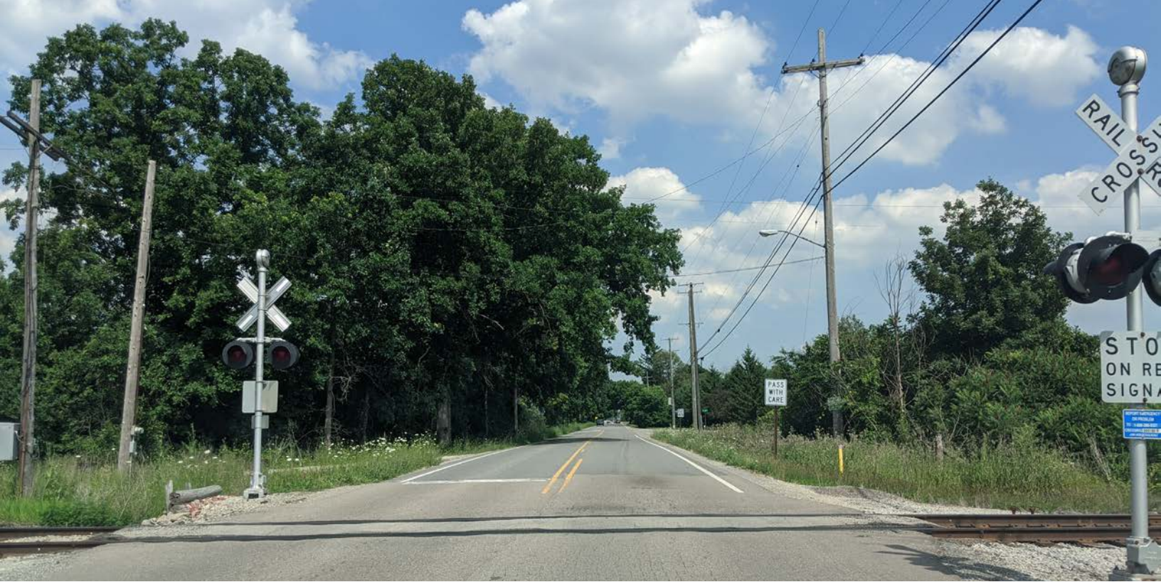
WILLIS RAIL CROSSING
